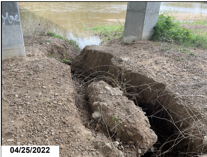
4' 8" deep ditch cut between columns #3 and #4 at bent #2. No footings are exposed.
