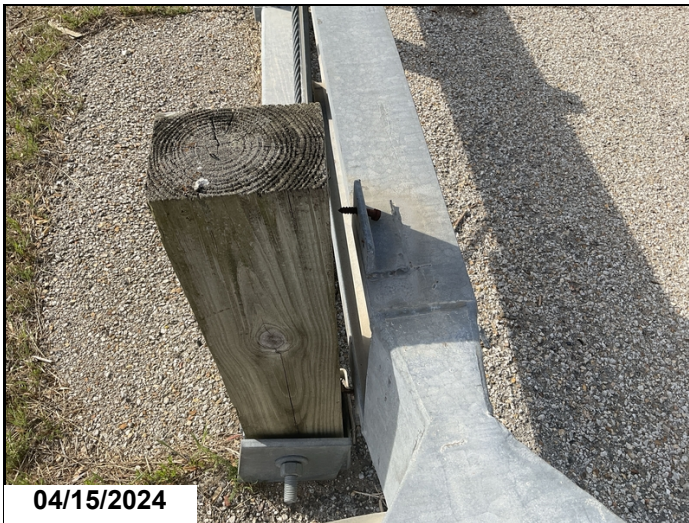
Left beginning end treatment is unattached to post.
