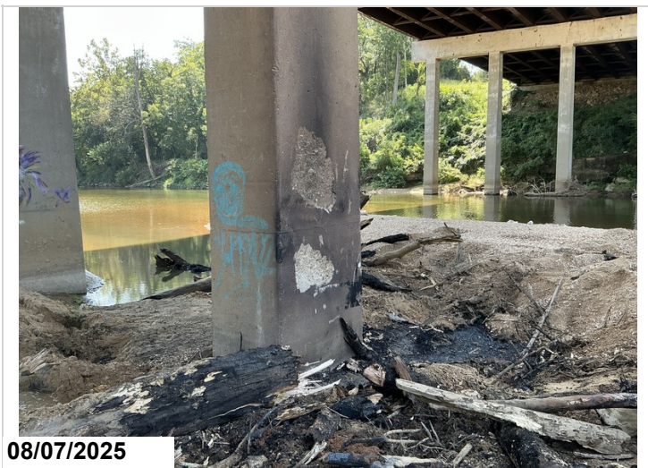
Bent 3, column 4 spalling and discoloration due to drift pile being burnt.
