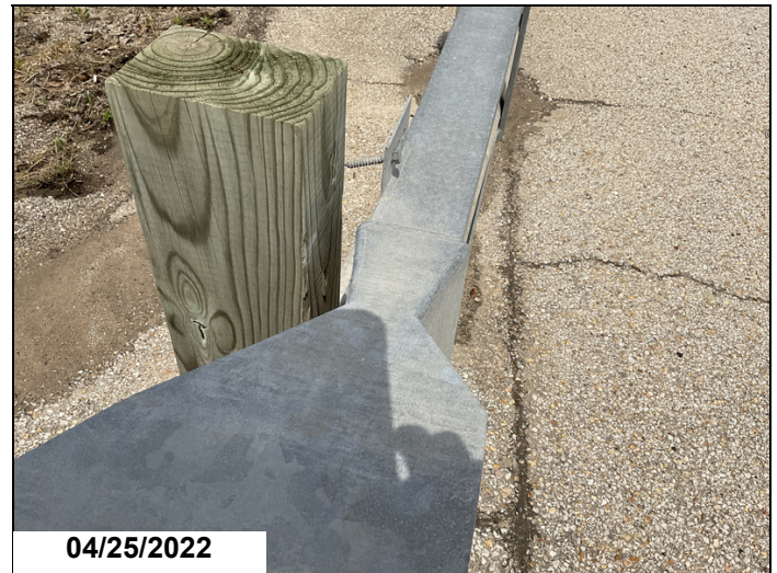
The right ending approach rail termination is not attached to the post.
