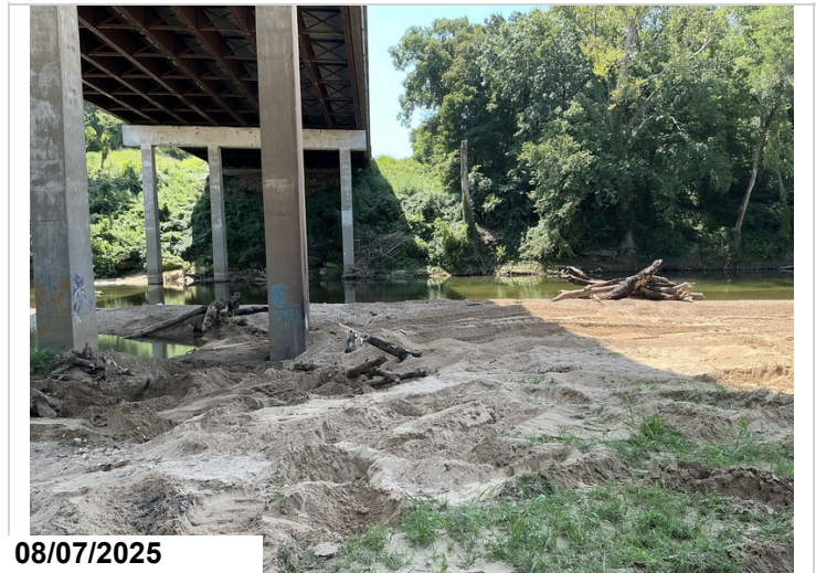
Remaining drift has been removed away from bent.
